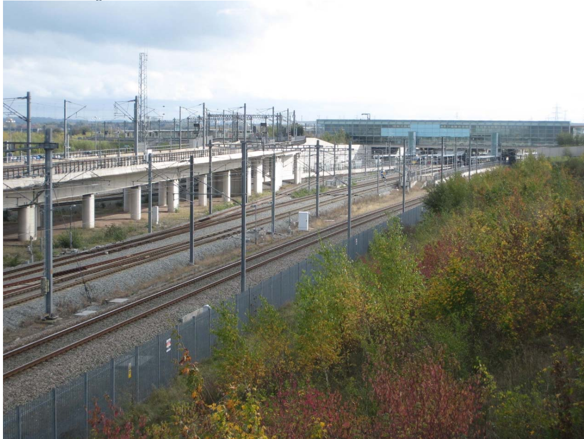
Photo 9. Looking toward Ebbsfleet International Station from the site.
